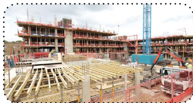
Construction work in Ocean Estate in Tower Hamlets.
